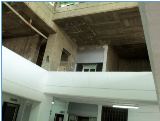
In Esmeraldas (MMI VI), a three-story reinforced concrete-frame/shear wall city government office building suffered minor brick infill partition damage. The building appears to have adequate sized columns and beams.
