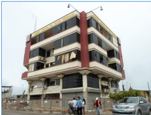
A five-story concrete city government office building in Pedernales (MMI VIII) suffered extensive damage to brick infill walls and window glazing.
