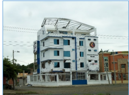
A five-story concrete city government office building in Pedernales (MMI VIII) suffered extensive damage to brick infill walls and window glazing.
