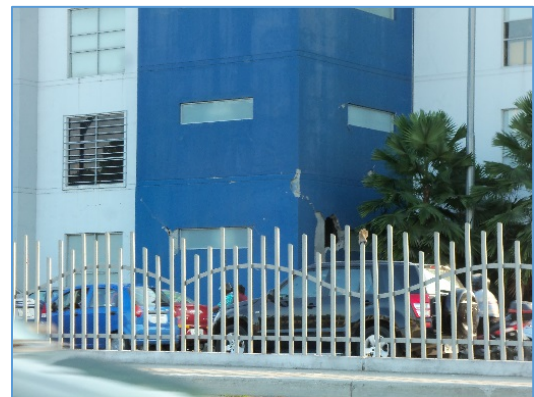
In Esmeraldas (MMI VI), a three-story reinforced concrete-frame/shear wall city government office building suffered minor brick infill partition damage. The building appears to have adequate sized columns and beams.
